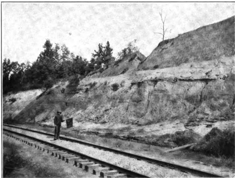
A. CUT AT CURVE, TENN.
